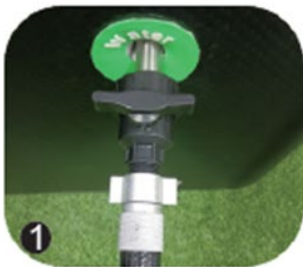
1 Close the shutoff valves on the inlet and outlet of the tub
