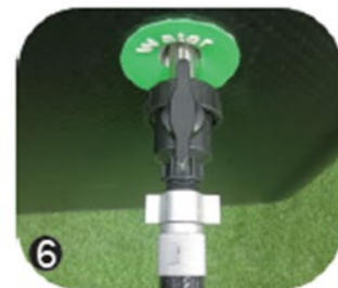
6 Open the shutoff valves on the inlet and outlet of the tub
